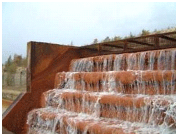
Figure 8-20: Aeration Cascade for Oxidation of Coal Effluent (88)
